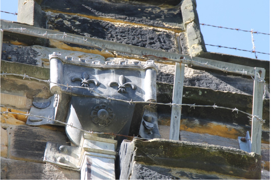
This 18 th Century lead hopper is protected by barbed wire which looks awful but does the job!
