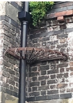
This lightning conductor is fitted with a protective sheath.
