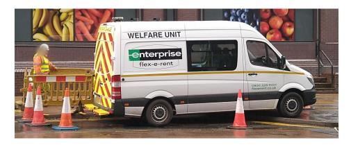
CDM in action: The worker has access to welfare facilities in the van. The site is clearly defined and measures have been taken to protect the public from the site (a hole in the pavement surrounded by fencing) and the worker is protected from traffic by the road cones.
